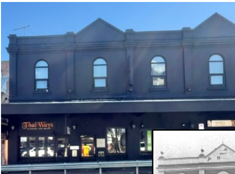
Albion Public Hall built 1887
